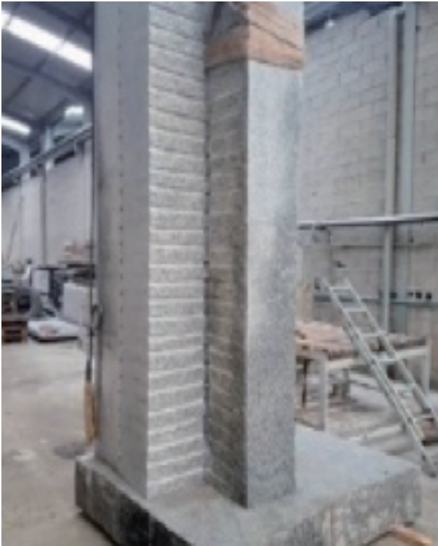
Fig. 1. Work in progress on the Cambridge Rules sculpture (UK). Source: www.cambridge.gov.uk
